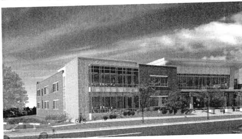
A rendering of the planned Madison College South Side campus at 801 W. Badger Road. PLUNKETT RAYSICH ARCHITECTS LLP
